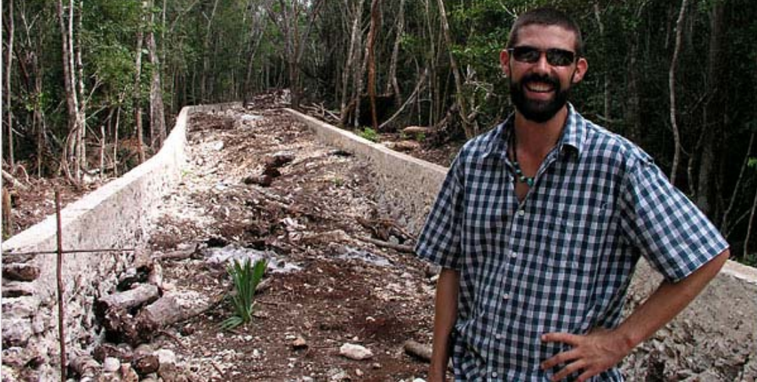
Matthew Schnurr, at the construction entrance to Los Árboles Tulum, 7.5 miles inland from the Caribbean coast.
